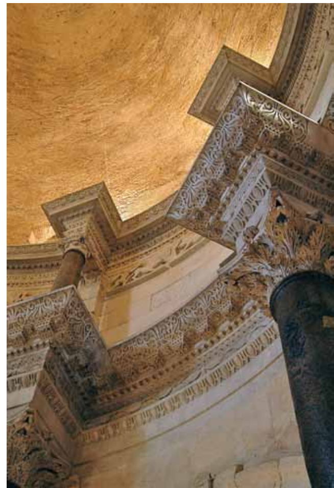
ABOVE The ornate decoration beneath the cupola inside the Mausoleum.
